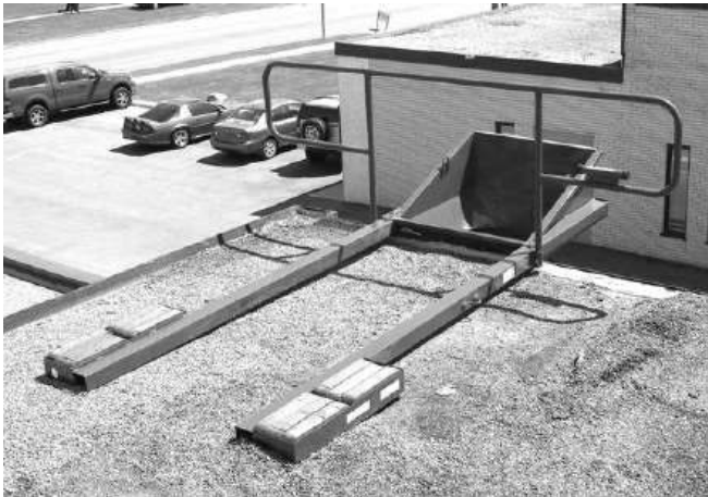
Trash Hopper Counterweight System
